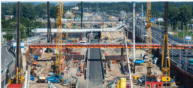
Gaasperdammertunnel under construction.
