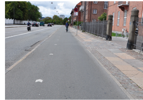
Creation of a right-turn lane with no traffic light (Copenhagen)
